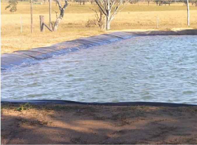
**A damp 'tide line' shows how close this pond is to overflowing, and there is nothing to prevent spillages from flowing directly into an adjacent drainage line/gully, and on to creeks and rivers.**
