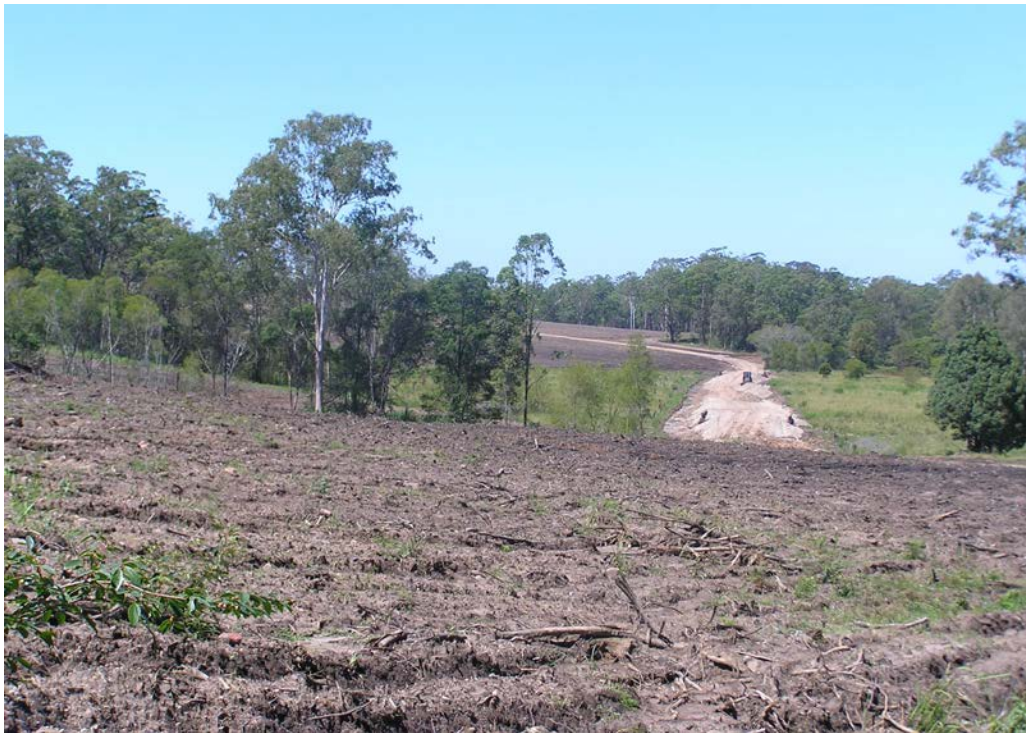
The clearing continues on.
