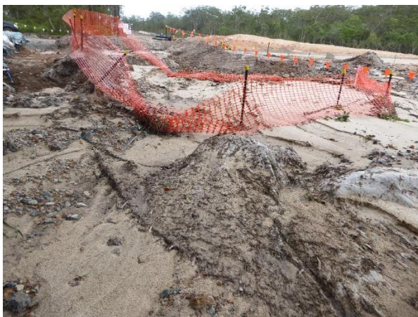
Barriers and booms washed away, and the wetlands swamped under tonnes of silt as the Pacific Highway upgrade took place. It took 6 years to complete and this type of incident was repeated time and again all along the 80km route through the Clarence valley. All can be blamed on ineffective erosion control.
