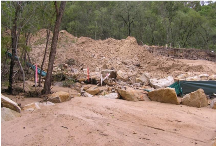
More ineffective silt trapping and more creek and river pollution from the construction of the access road to the Shannon Creek dam
