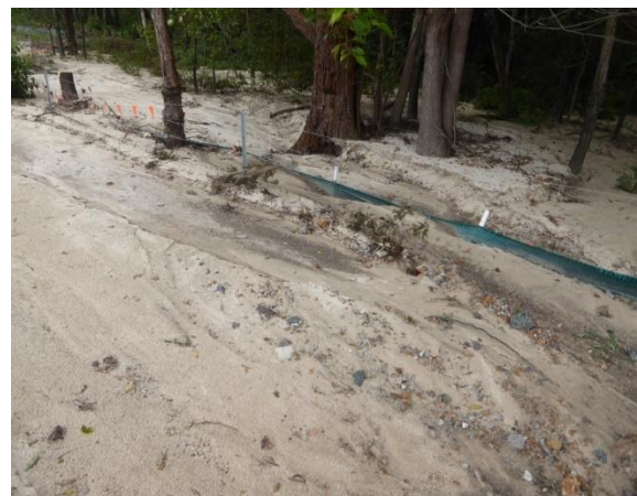
Barriers and booms washed away, and the wetlands swamped under tonnes of silt as the Pacific Highway upgrade took place. It took 6 years to complete and this type of incident was repeated time and again all along the 80km route through the Clarence valley. All can be blamed on ineffective erosion control.
